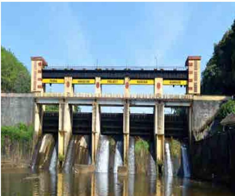
The Pamba Irrigation Project consists of a barrage at Maniyar across Kakkad River, a major tributary of Pamba. The river Kakkad originates from Kakkiar Malai, flows in a north-western direction and joins Pamba at Perinad. The project aims at the utilization of the firm discharge of the tailrace water of Sabarigiri Hydro Electric Project for Irrigation purposes, which let the tailrace water into the river Kakkad and is picked up at Maniyar by a barrage situated at 9° 20' N and 76° 53' E.
