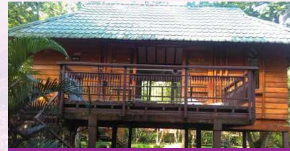
Cottages - Renovation works - Kottayam
