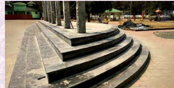
Padinjarekkara Beach - Entrance area & Toilet block- Malappuram
